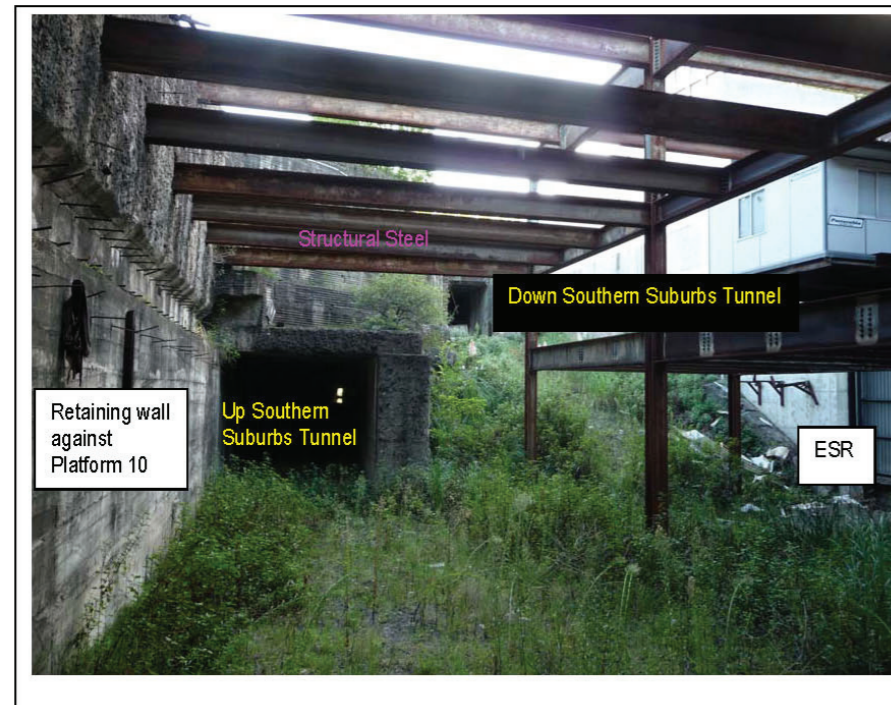
Image 1 – Void between Platform 10 and Eastern Suburbs Railway looking towards Sydney
